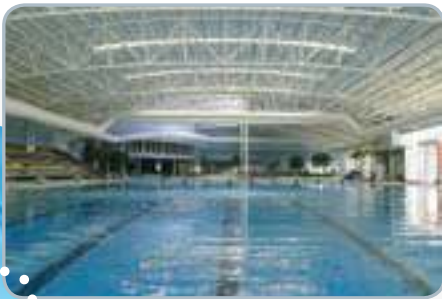
Bunbury Leisure Centre, WA, Australia AVP Constructions*
